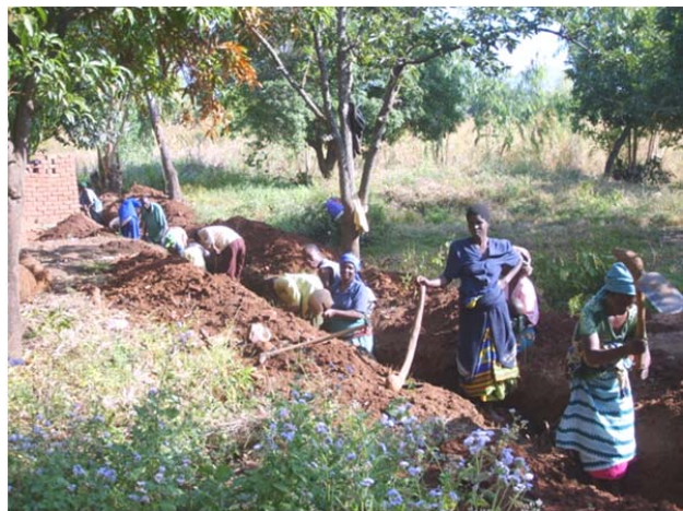
Figure 2:3 Community members participating in trench excavation
